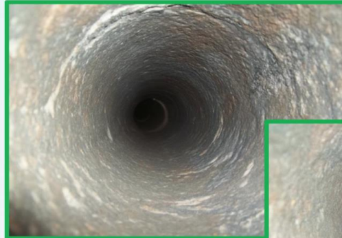
Bitumen liner being removed
