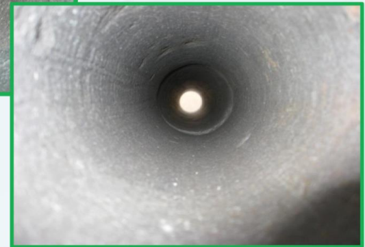
Fully prepared for liner bonding
