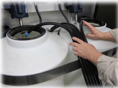
Grout hose recirculation when necessary
