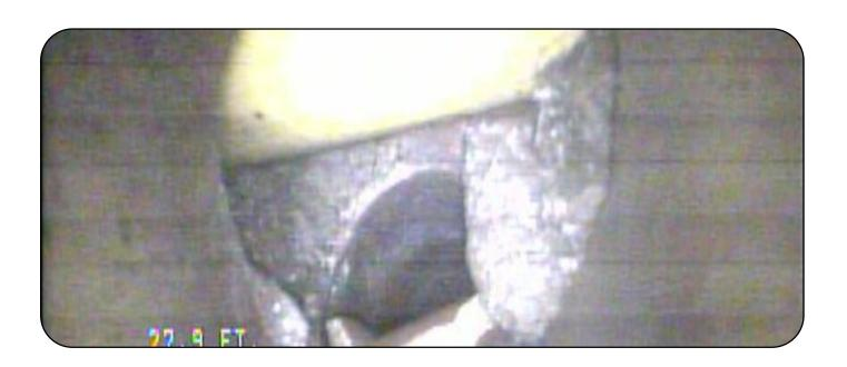
"In the St. Paul explosion, a sewer contractor punctured a natural gas line that he didn't know had been inserted through a sewer pipe, a procedure called a cross bore. The line break caused gas to leak into a house on Villard Avenue in the Highland Park district, sparking an explosion."
