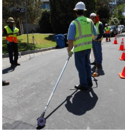
A long-handled, air-powered grinder with plastic abrasion disk was used to prepare the pipe surface for wire bonding.
