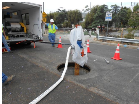
Ready to launch. The fire hose provided water to push the tool to the far end of the main. A plastic sheet contains water that leaks from the assembly. The hydrant is braced to the trailer to counteract the winching force.
