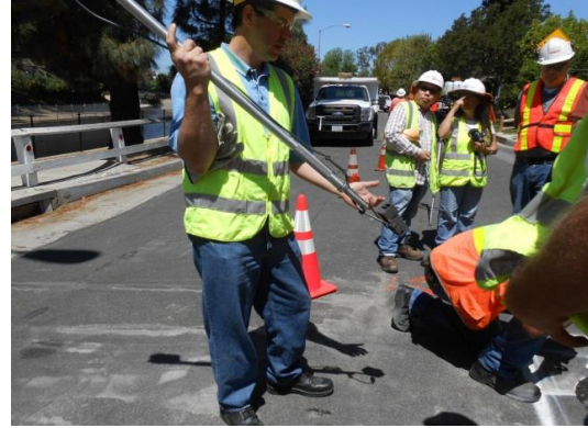
Another long-handled tool was used for exothermically welding the anode to the pipe. 1
