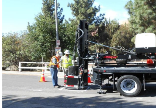
The coring rig positioned over excavation location.
