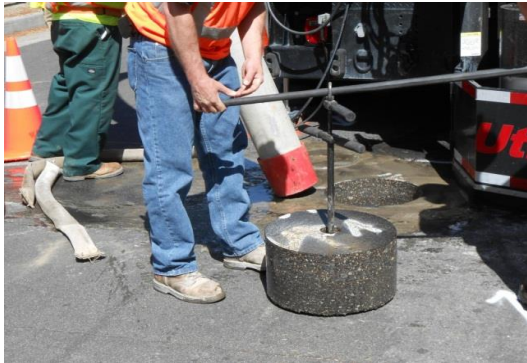
Two persons lifted the core using a special tool that grips the center pilot hole. The core was then tipped on its side and rolled out of the way.
