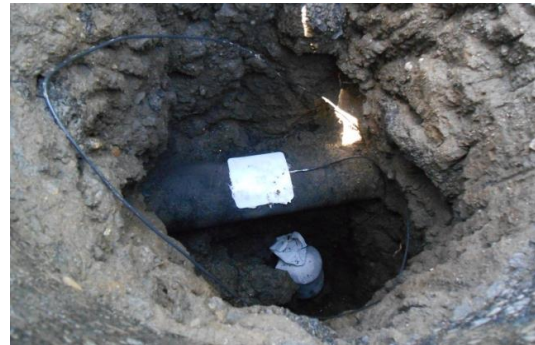
Another long-handled tool was used for exothermically welding the anode to the pipe. 1
