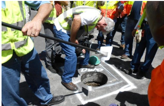
A long-handled, air-powered grinder with plastic abrasion disk was used to prepare the pipe surface for wire bonding.
