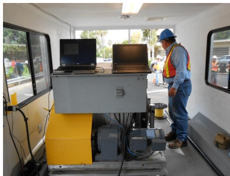
The location of the NDE tool is tracked by measuring the amount and speed of tether rope used deployment. Underneath the table is the motor used to winch back the tool. All tools and equipment were powered from a small electrical generator.
