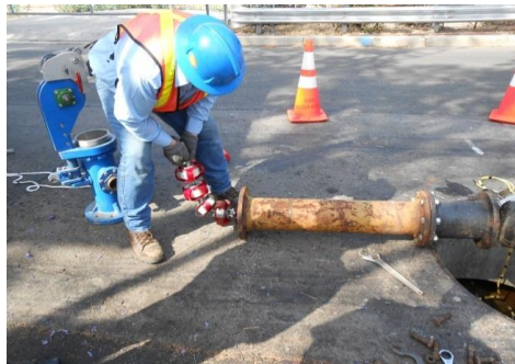
Inserting the tool into the launching port. Normally this tool is launched from a fire hydrant's vertical drop leg.
