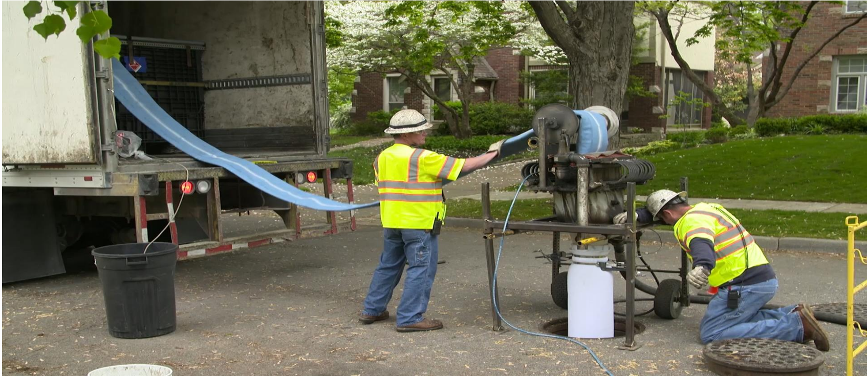
CIPP with Steam Curing -- Source: Insituform Technologies
