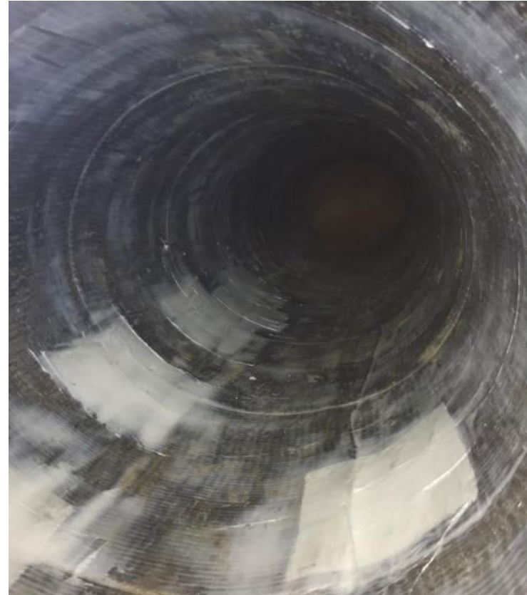
Completely Installed FRP System
