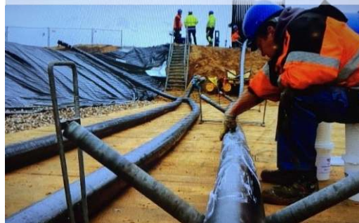
Cable pull-in lubrication
