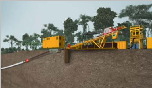
► Horizontal Directional Drilling
