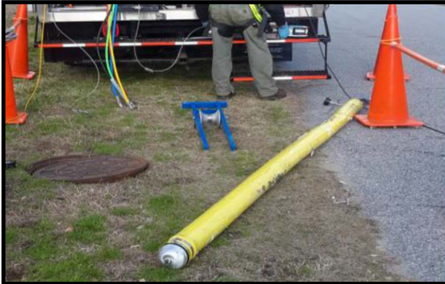
Grout Packers for longitudinal cracks
