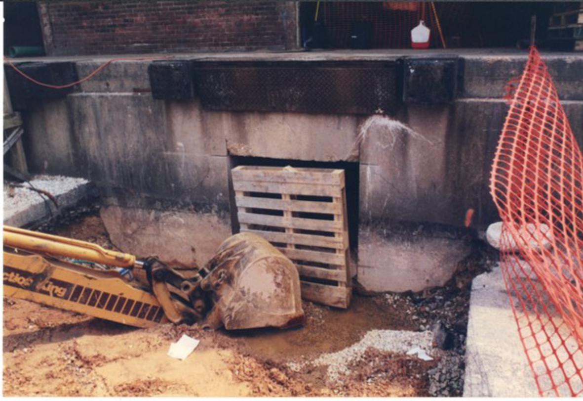
CUT ACCESS WAY THROUGH FOUNDATION GRADE BEAM
