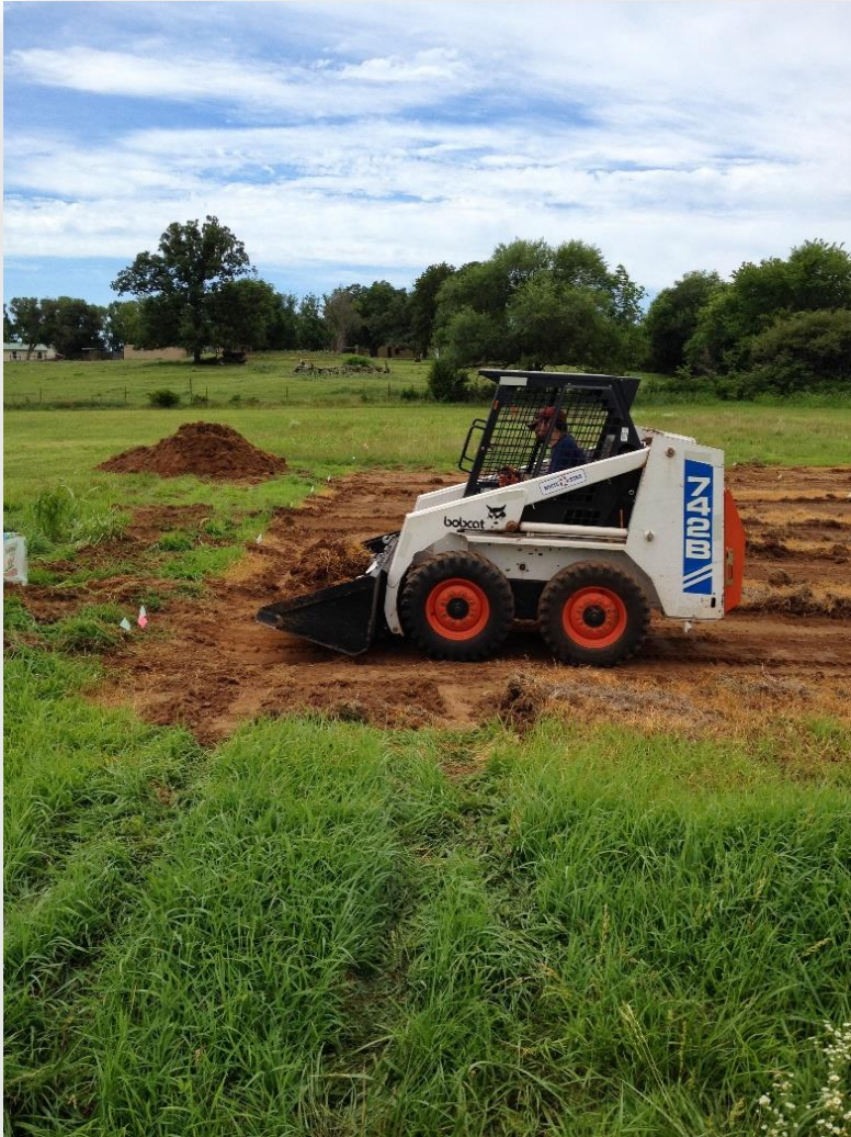
Plots Scraped Clean and Levelled
