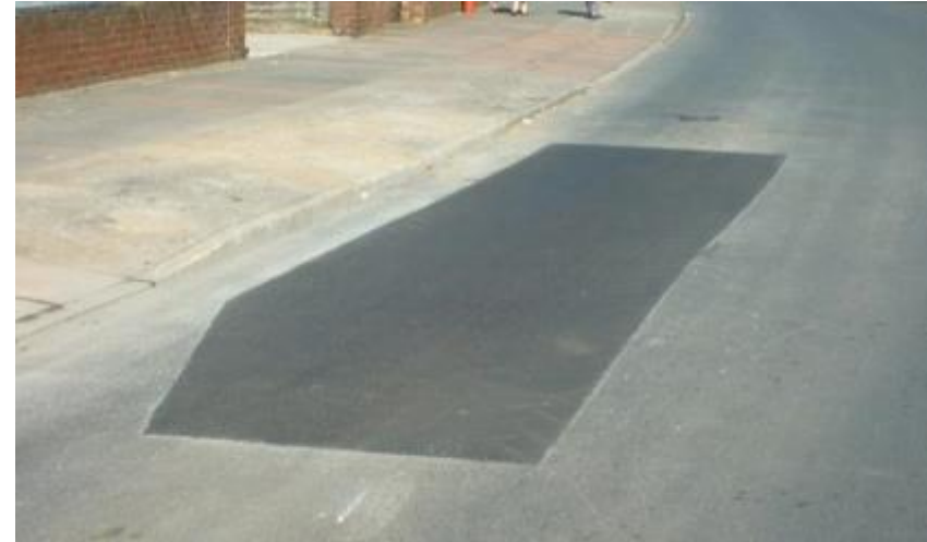
Backfill excavation and permanently re-instate.
