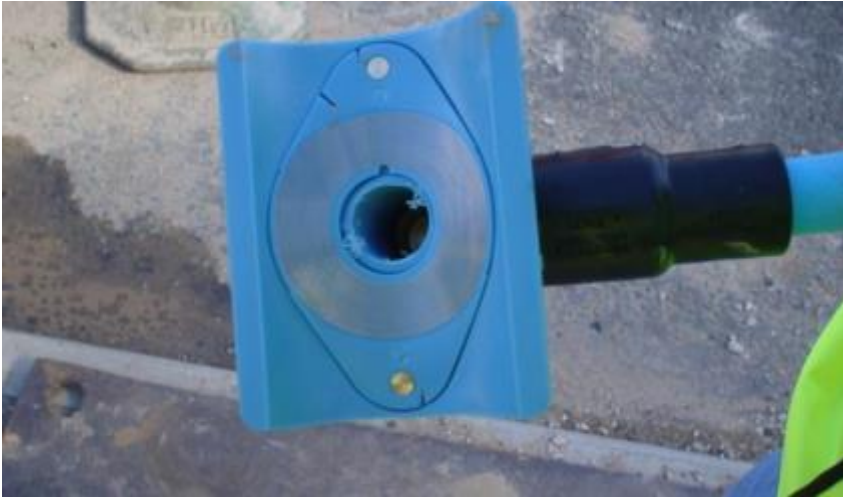
Install electro-fusion saddles for service connections.
