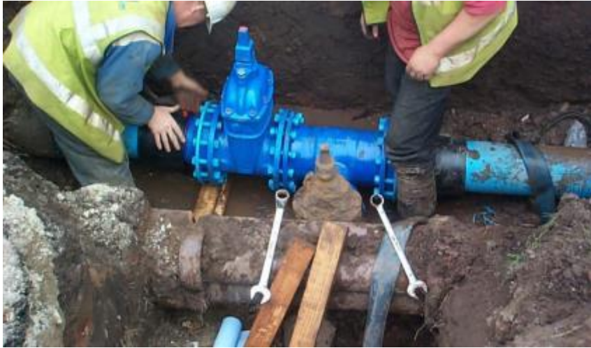
Install necessary branches, valves and hydrants.
