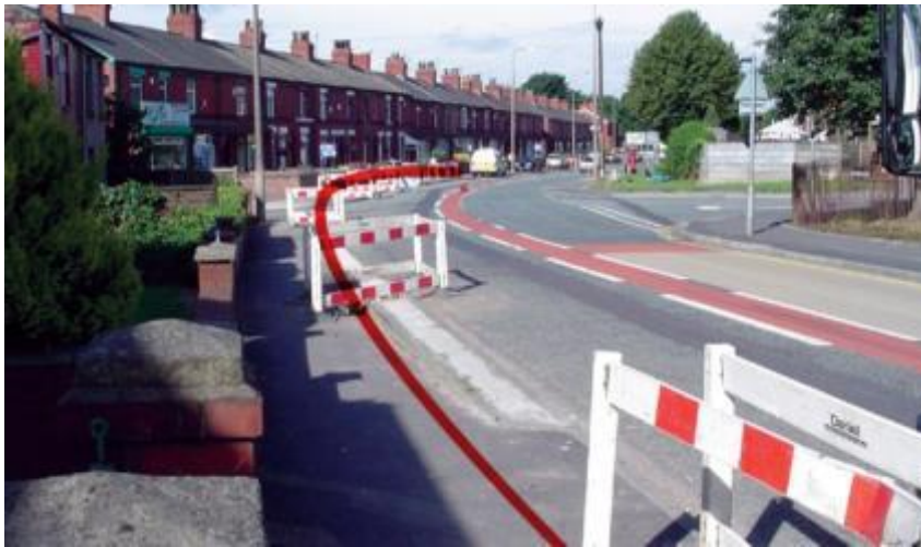
Excavate launch, reception and service pits.
