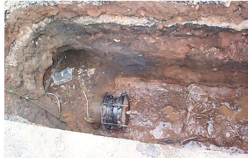
Cut existing cast-iron main, install cap end and secure. Re-establish supply to existing main.
