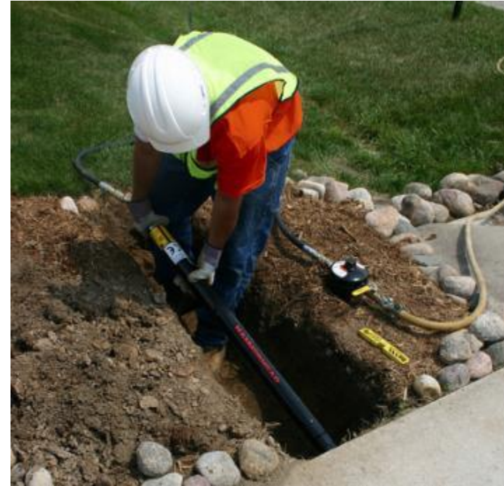
Pneumatic piercing tools used for installing new services.
