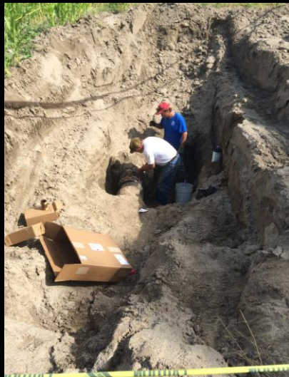
Install Hot Taps
