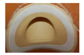
• A bladder is used to inflate to put in place the resin saturated liner
