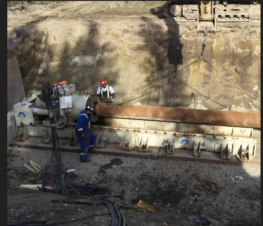
INSTALL MULTIPLE LENGTHS OF STEEL CASING TO MAXIMIZE PRODUCTION
