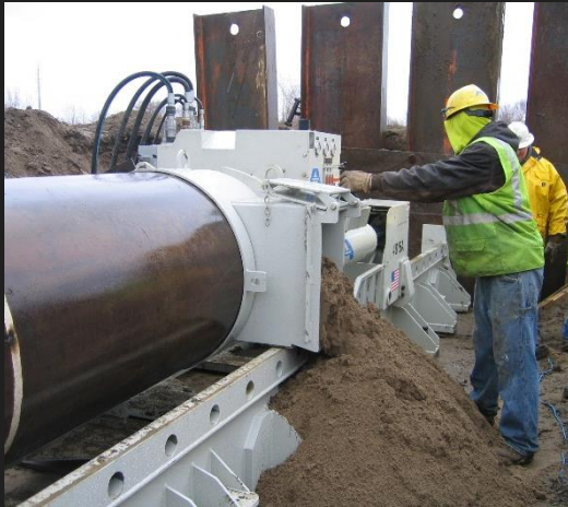
CASING ADAPTER TO DISCHARGE SOIL VOLUME
