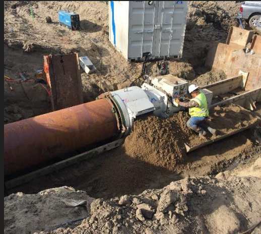
MASTER PUSH RING ADDS ADDITIONAL TORQUE FOR LARGER DIAMETERS AND LONGER DRIVES
