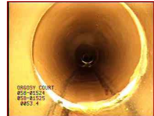
Sewer Pipe in Baton Rouge area after CCTV Cleaning
