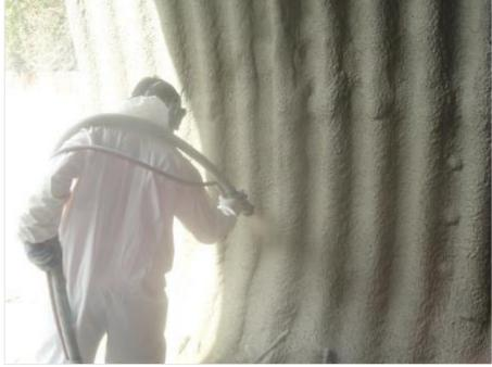
The material was applied on the sides and then across the crown of the structure
