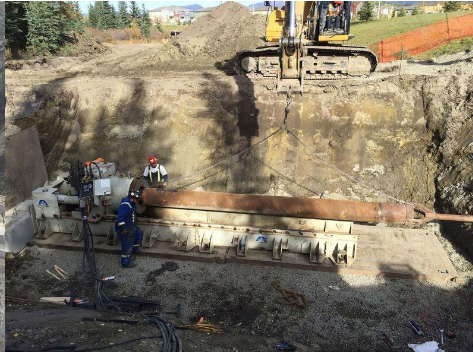
Machine Capable of Auger Boring up to 36" Steel Casing with standard adapter.
