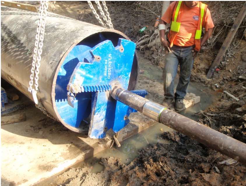
Guide Rod Swivel-Simple-Ideal \leq 24'' Diameter and <200'
