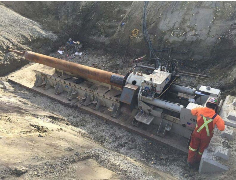
4800 Series GBM with 36" Auger Boring Master Pusher Attachment.
