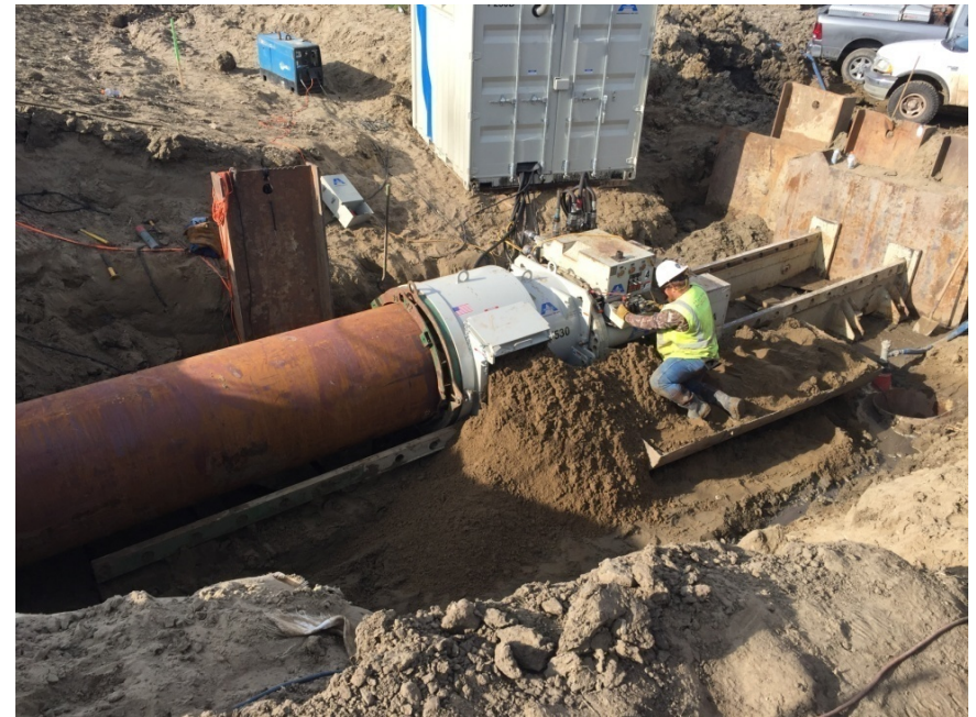
48" HTCA-Shown Jacking 40" Casing
