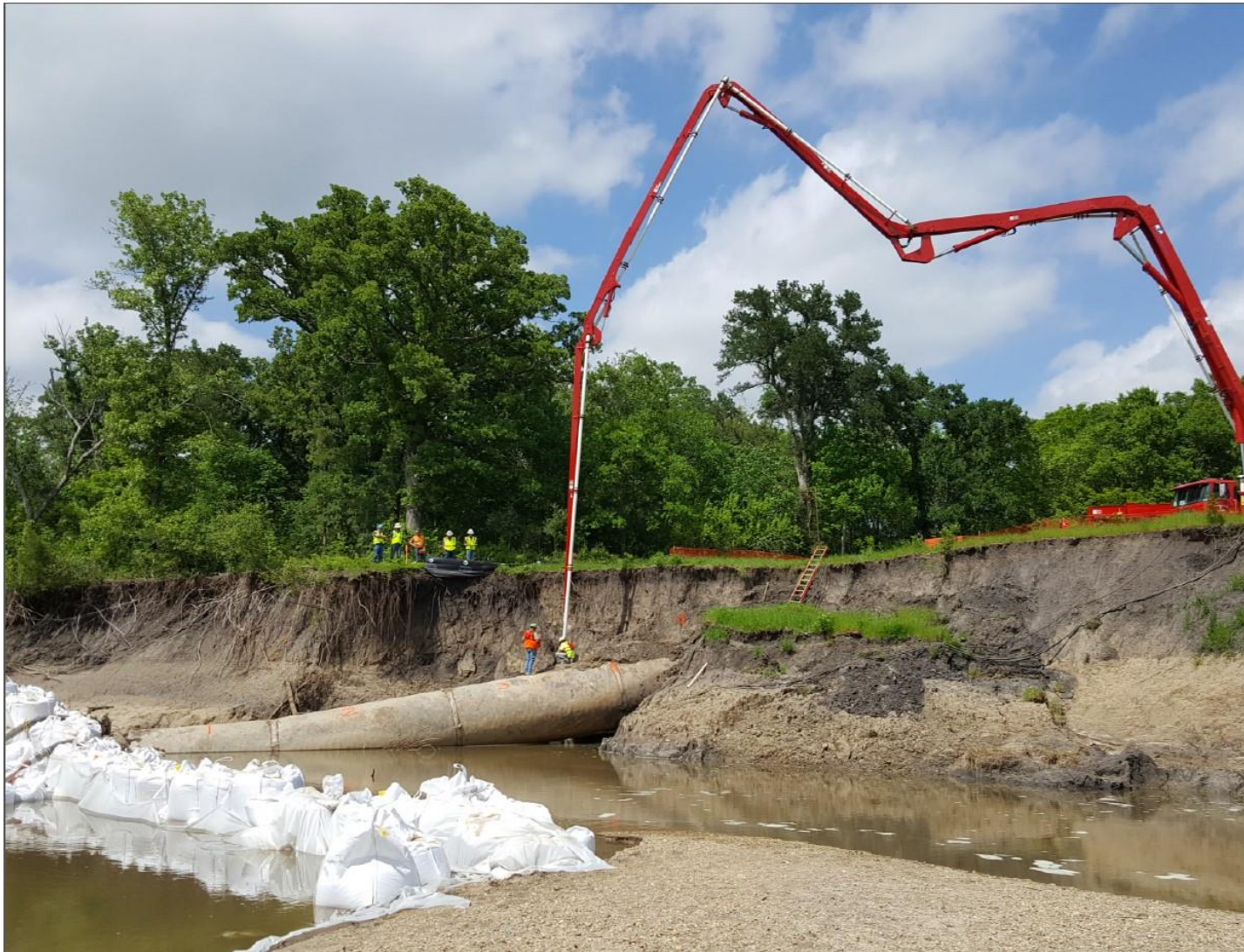
Pipe Stabilization
