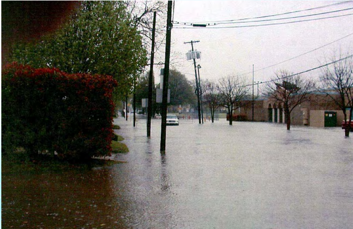
Worth Street Flooding
