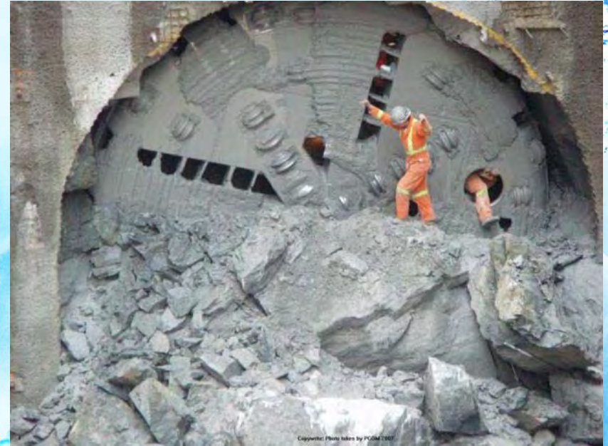
Workers on a TBM after break-through
