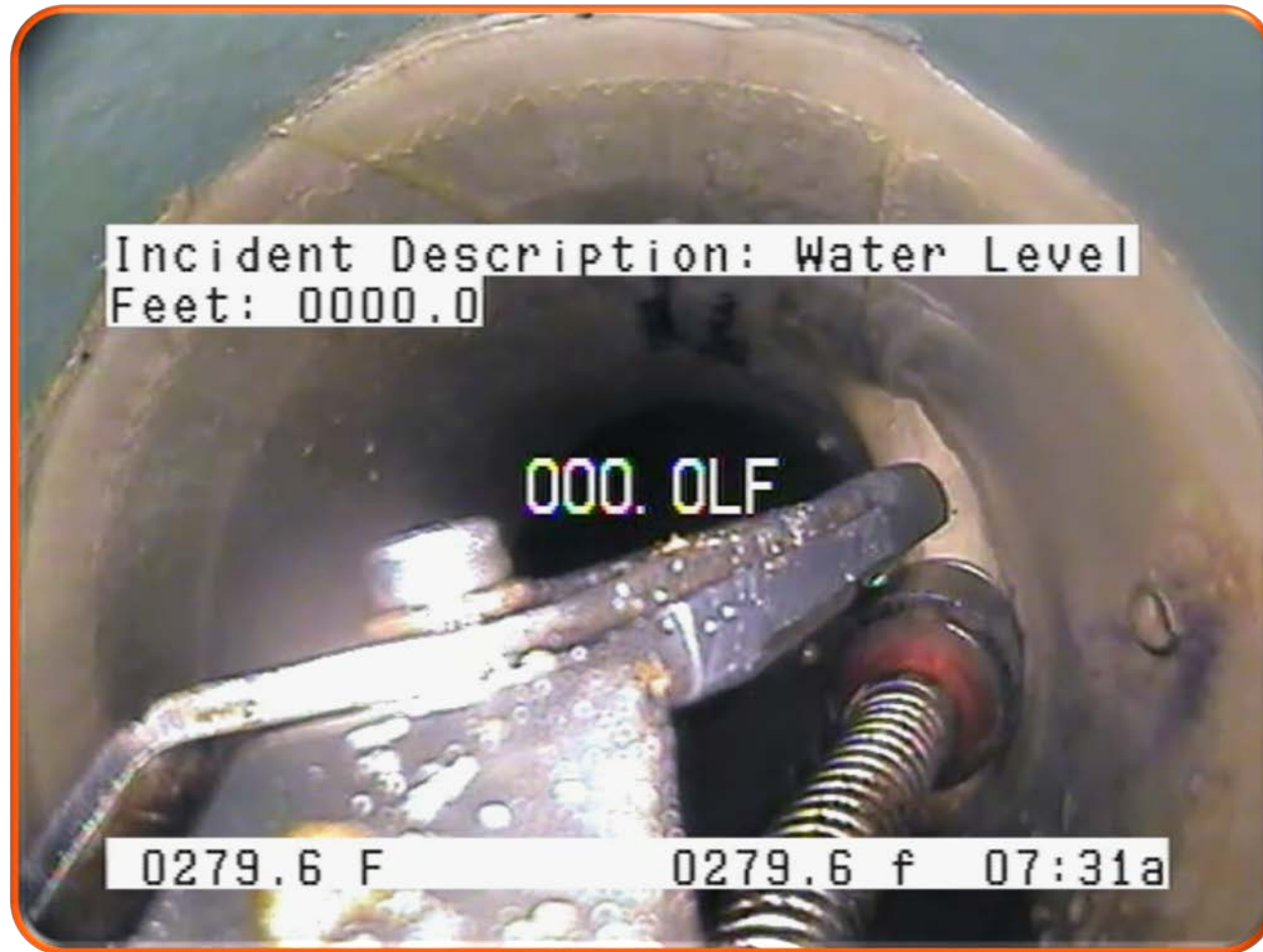
Collection System After Mainline and Main to Lateral Rehabilitation Installation and Post Installation Video performed by Musson Bros., Inc., Brookfield, WI
