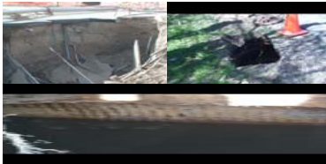
Pipe Collapse- Excessive Corrosion = ADDITIONAL 1.5 million dollars ER
