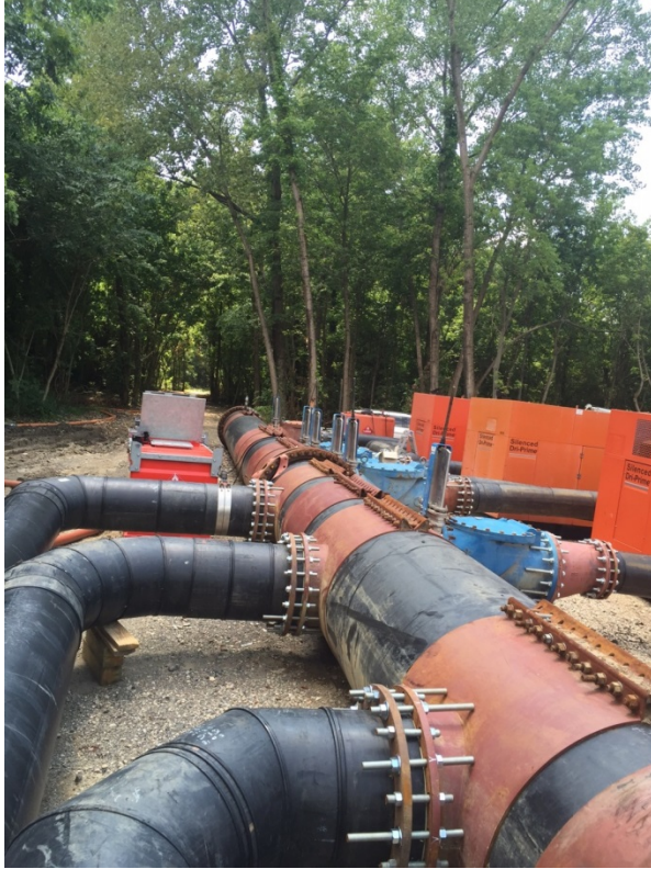
The manifold with discharge pipes, which would travel to the discharge point, 3,500 feet away.
