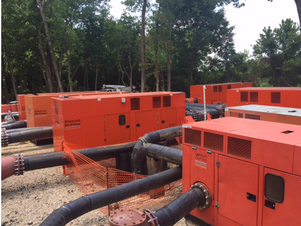
The bank of diesel-driven critically silenced CD400M pumps, in place for the Mud Island bypass.
